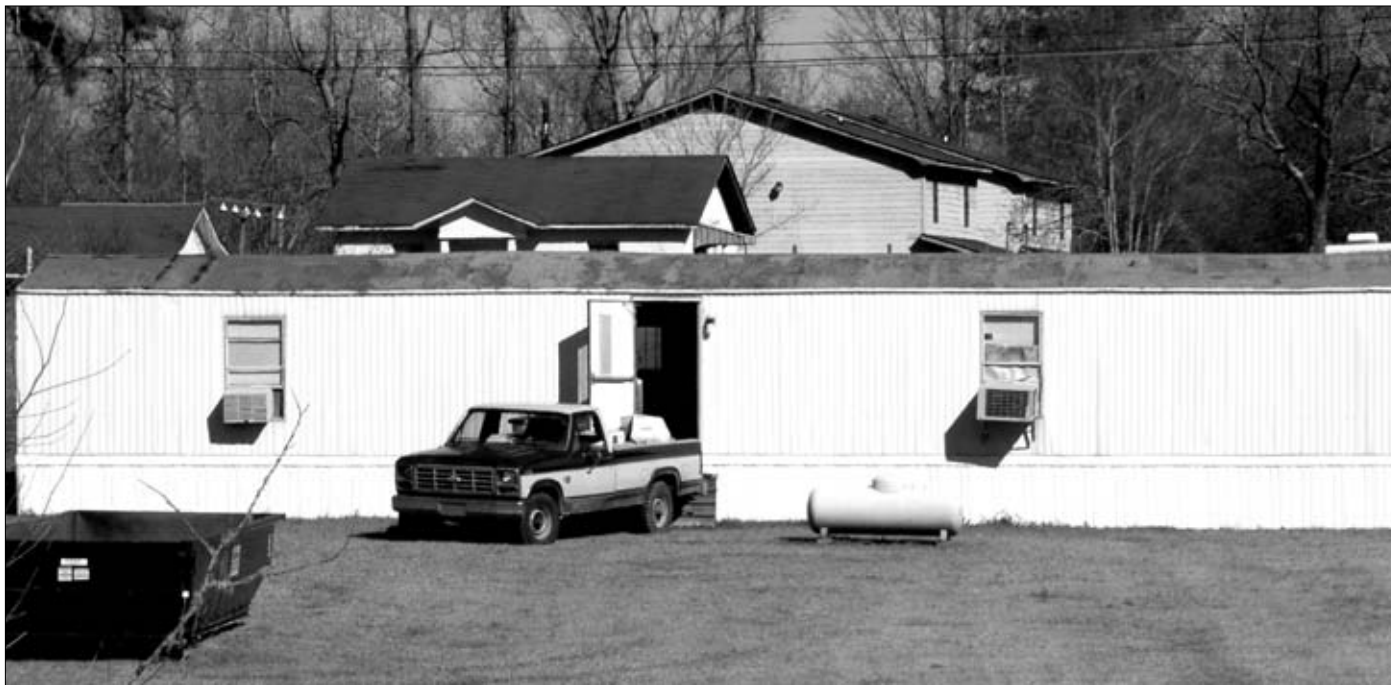
Work is in progress on what will become Alternative School for Choctaw County students. The mobile unit stands in front of the Board of Education office on Tom Orr Drive in Butler. Choctaw Sun photo by Dee Ann Campbell
